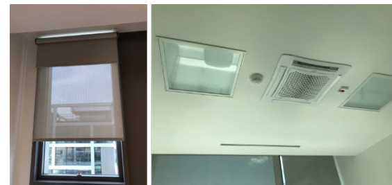
Fig. 2 – The double layer internal roller shades devices (left) and the lighting system installed in the three cabins (right)
