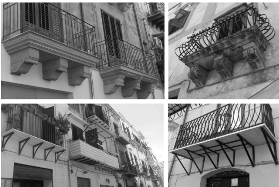
Fig. 2 – The main types of balconies. Stone balcony (on the top), metallic balcony (on the bottom) (picture by Zarcone Roberta, 2017)
