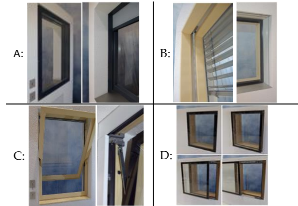
Fig. 4 – Opening/operation schemes of prototype A – D.
