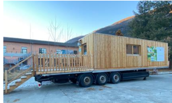
Fig. 2 - Prototype house made of hemp concrete and wood
