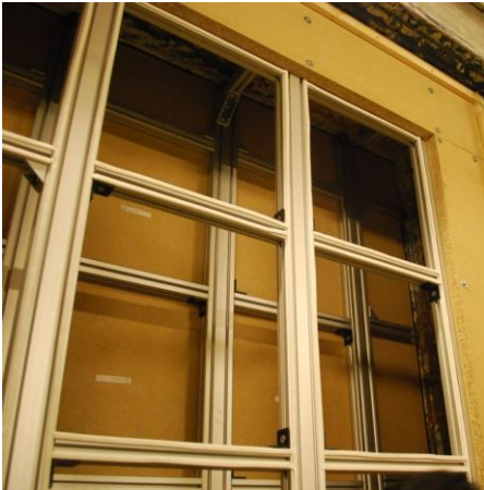
Fig. 1 – View of the experimental double-wall with the frame structure for the installation of flexible (individually removable) modular components.
