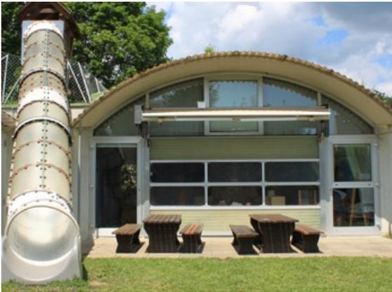
Fig. 5 – South facing wall with the large garage-type rolling door (pictures by the authors)
