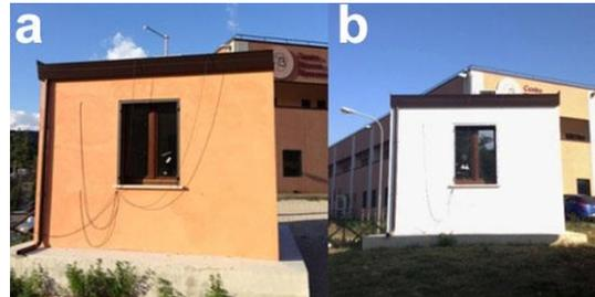
Fig. 1 – (a) Cool and (b) standard configuration of the case study building
