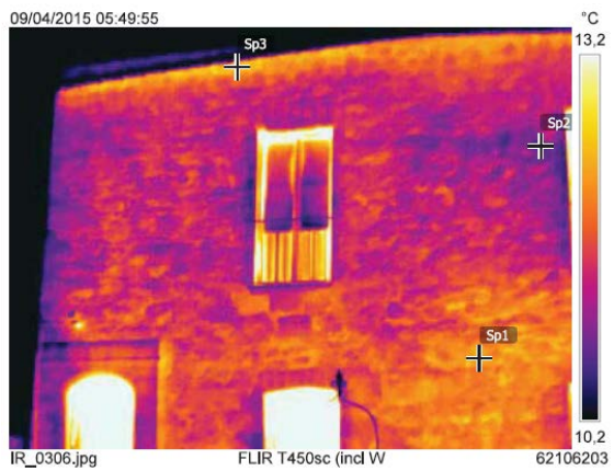
Fig. 7 – IR of the main North facade
