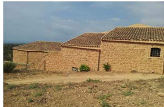
Fig. 1 – South view of the building
