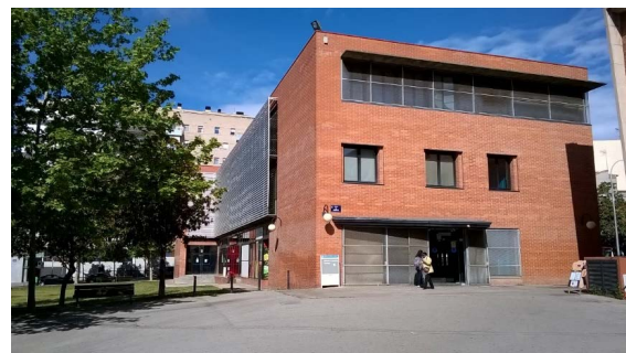
Fig. 1 – The south east façade of the UPC Terrassa library building
