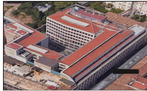
Fig. 1 - The case-study building (Google Earth)
