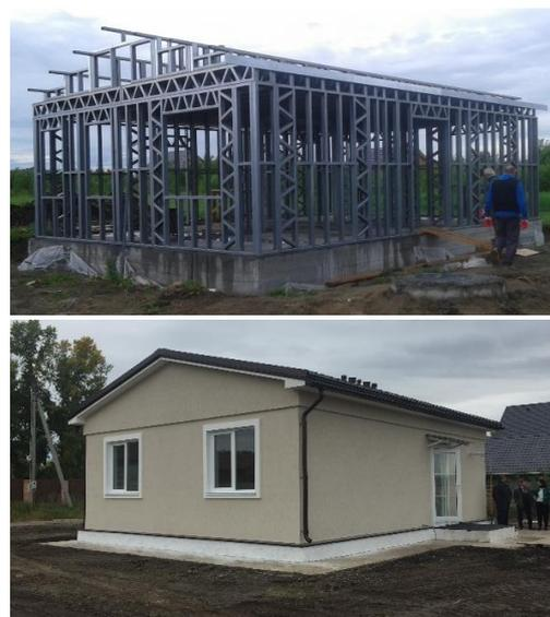
Fig. 1 – The building during (a) and at the end of the construction phase (b). Picture by Giovanni Manzini, 2019
