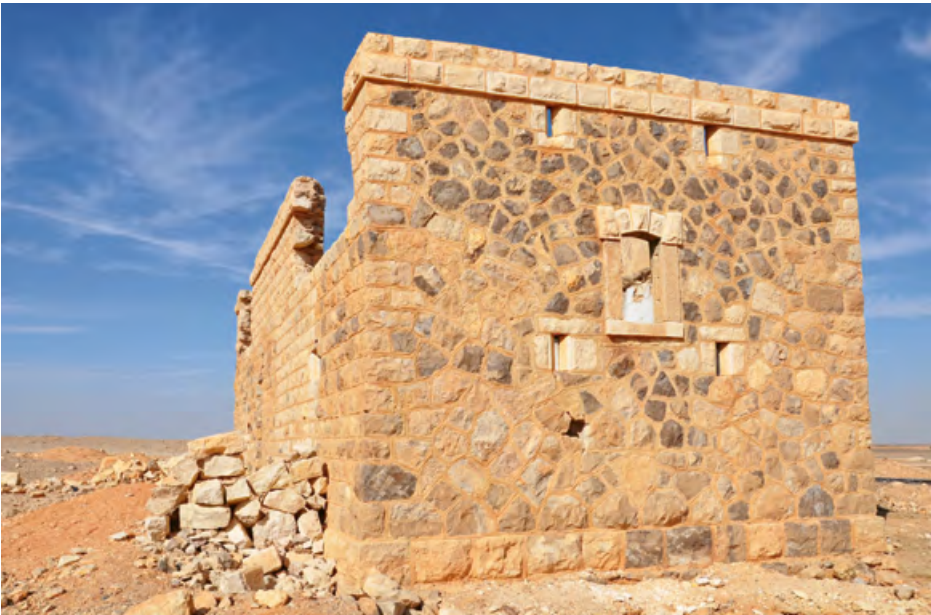
7 The Blockhouse, Turkish railway strongpoint showing signs of original 1905 construction, 1918 war damage, and 1960s refurbishment, Jordan. © Nicholas J. Saunders.
