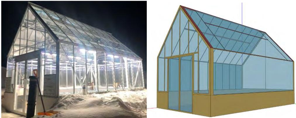
Fig. 1 – (a) Experimental small-scale greenhouse and (b) Building energy model (BEM)
