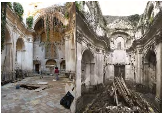
Fig. 2 – Internal view before the restoration works
