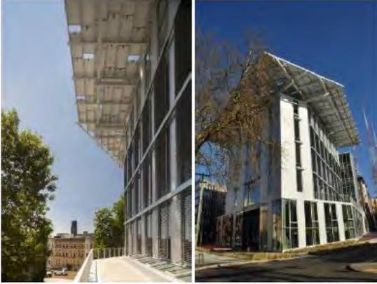
Fig. 2 – Views of the existing Bullitt Center, focusing on the integrated shading louvers and the roof with its shadow
