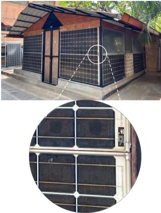
Fig. 1 – End-of-Life Photovoltaic panel integrated building with noticeable source of thermal bridging at the edges
